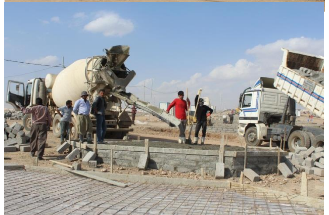
Ongoing construction at Khanke IDP camp, Dohuk governorate. UNHCR/G. Gubaeva.
